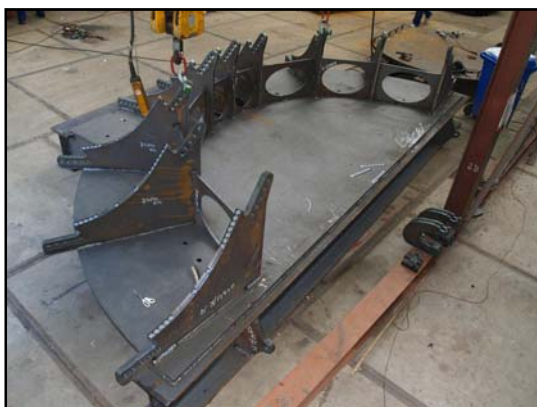
Figure 9. Assembly jig for panels comparable to ITER panels
